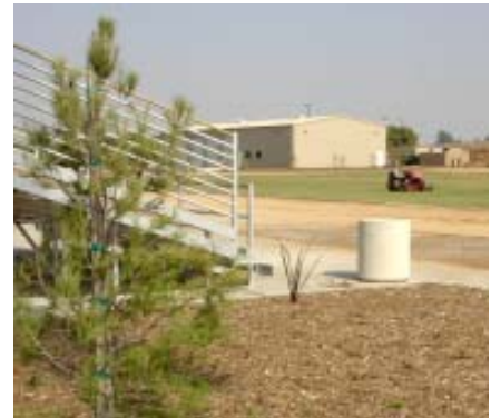
Bleachers await fans beside the new track and soccer stadium. In the background stands the new shop and bus facility.
